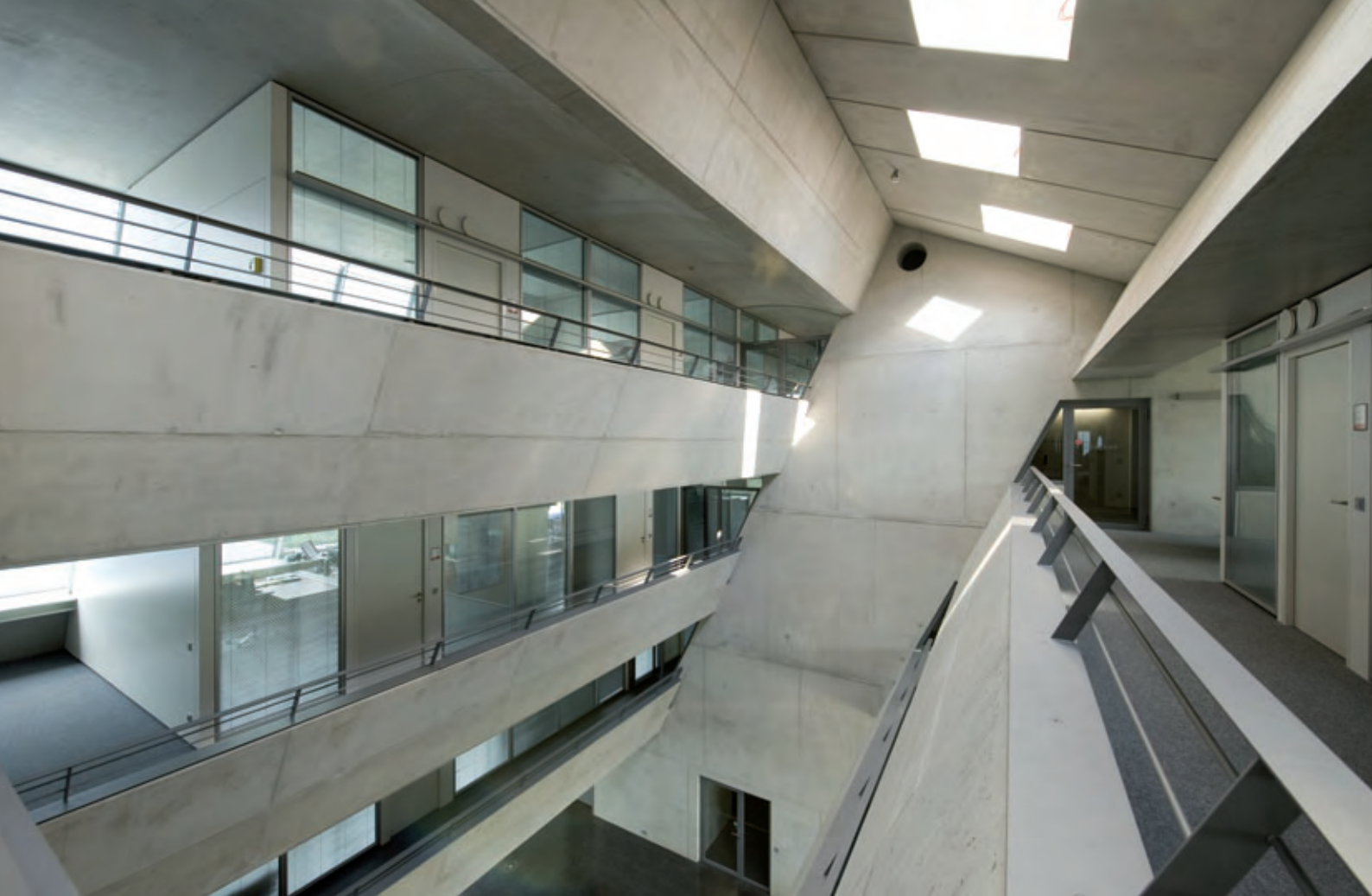
The building, which is inclined towards the south, uses non-dazzling daylight to a greater extent in the north and reduces the irradiance of heat into the building in the south by the use of the Fresnel effect.
